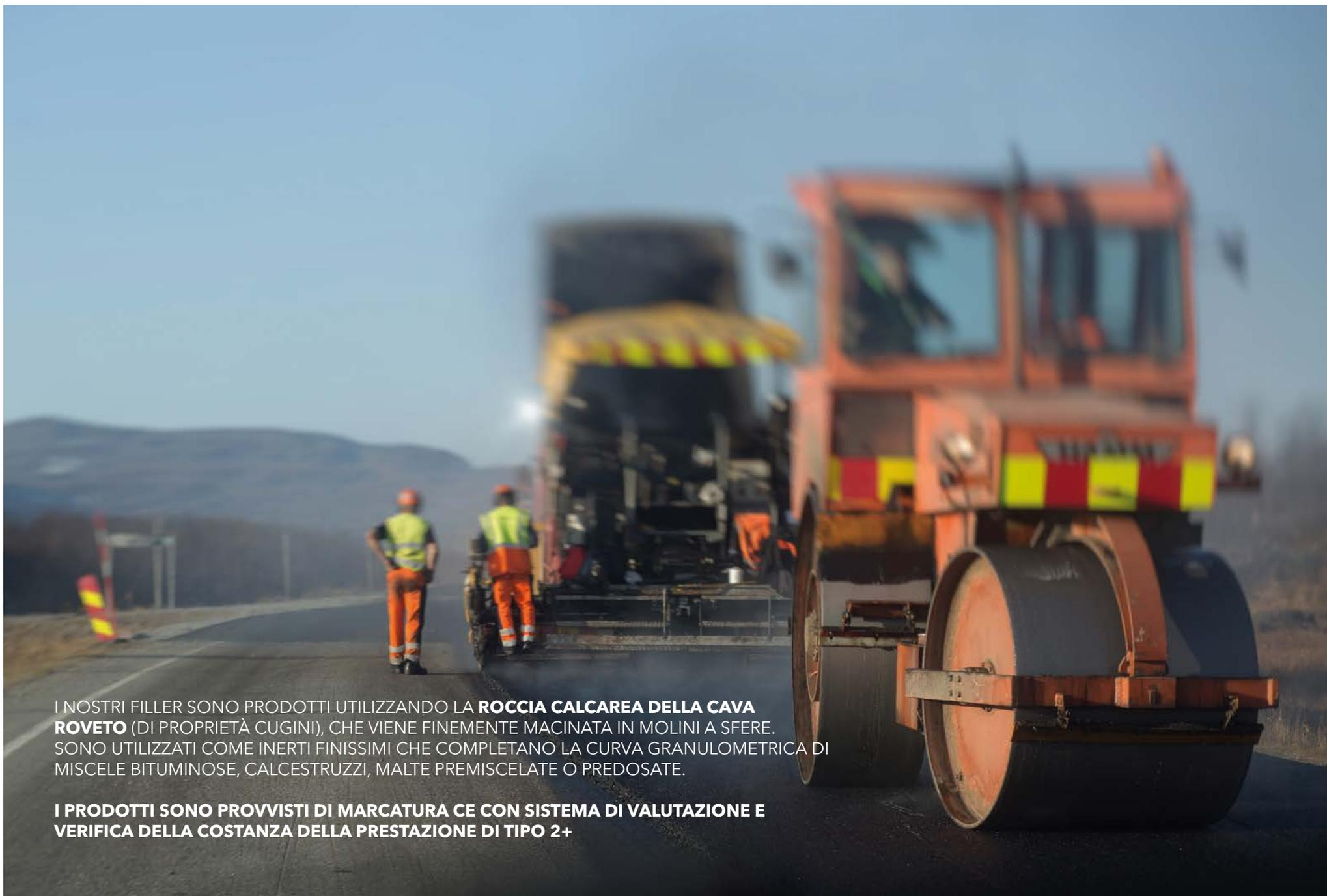
I NOSTRI FILLER SONO PRODOTTI UTILIZZANDO LA **ROCCIA CALCAREA DELLA CAVA ROVETO** (DI PROPRIETÀ CUGINI), CHE VIENE FINEMENTE MACINATA IN MOLINI A SFERE. SONO UTILIZZATI COME INERTI FINISSIMI CHE COMPLETANO LA CURVA GRANULOMETRICA DI MISCELE BITUMINOSE, CALCESTRUZZI, MALTE PREMISCELATE O PREDOSATE.
